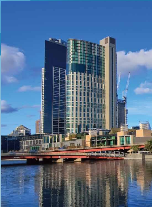
Crown Casino (Melbourne)
